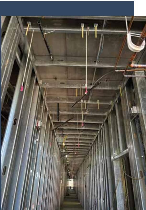
Interior Prefab Hallway
