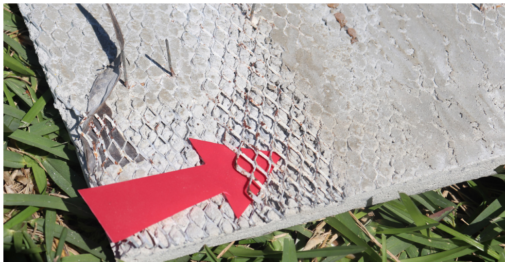
This image shows areas where the lath has been fully embedded on all sides by the stucco—as well as areas (red arrow), where the lath is fully free-floating, with no embedment. The areas where embedment is insufficient are prone to issues from moisture penetration and corrosion.
