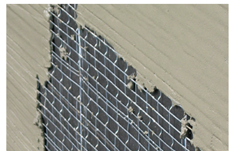
Welded wire lays down evenly with uniform furring.
